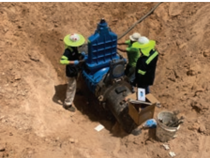
6 | Installing the bonnet
