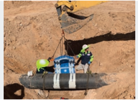
2 | Fitting the bottom (part B) of the AVT EZ Valve
