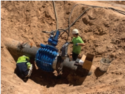
4 | Milling the 120° slot across the pipe
